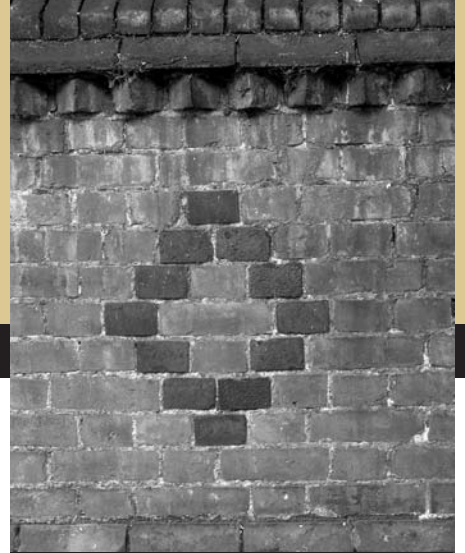
Wall along Grove Hill: decorative details are common throughout the area
