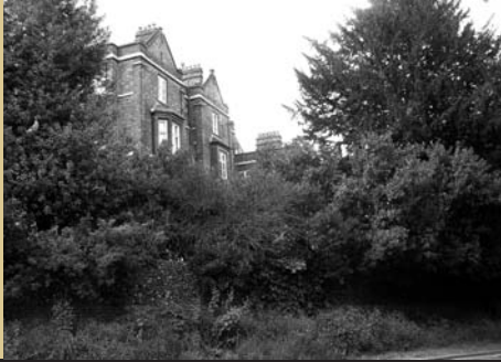
Rear of Boarding houses on Grove hill
